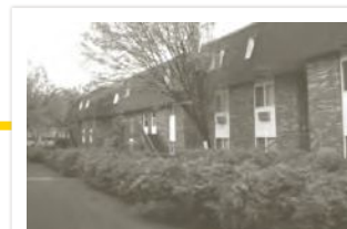
Briston Arms, Cambridge, MA: POAH preserves a 154-unit family apartment community in one of hottest real estate markets in the country
