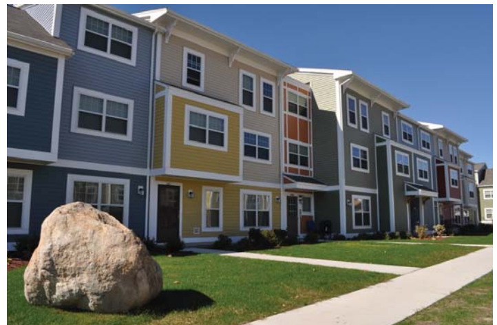
Photo: Courtesy of Preservation of Affordable Housing POAH used federal and state LIHTCs to rehabilitate and preserve United Front Homes, now called Temple Landing, in New Bedford, Mass.
