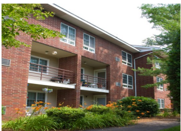
Bridle Path Apartments, Randolph, MA
