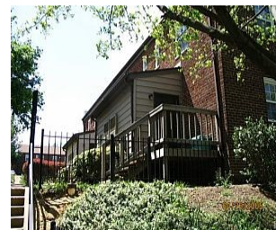
Garfield Hill Apartments, Washington, D.C.
